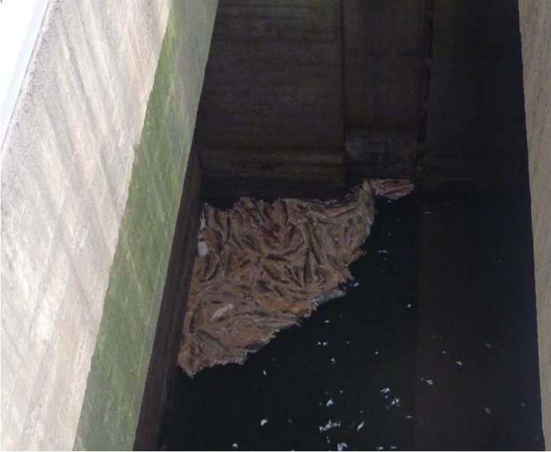
Figure 1. Unit 8 tail log slot from above, looking south.
